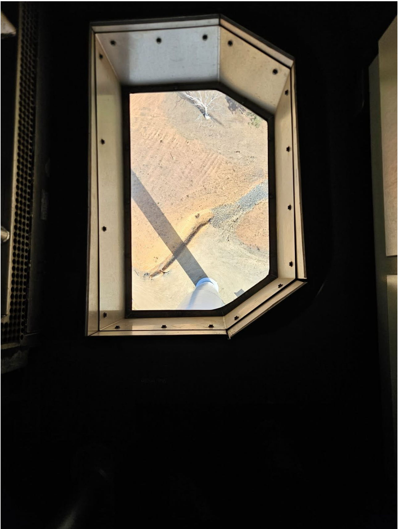
Figure 8: Hatch that Nankeen Kestrels were entering through the base of the nacelle at WTG 01. Image shows inspected hatch area where no nests or birds were present prior to making the turbine operational again.
