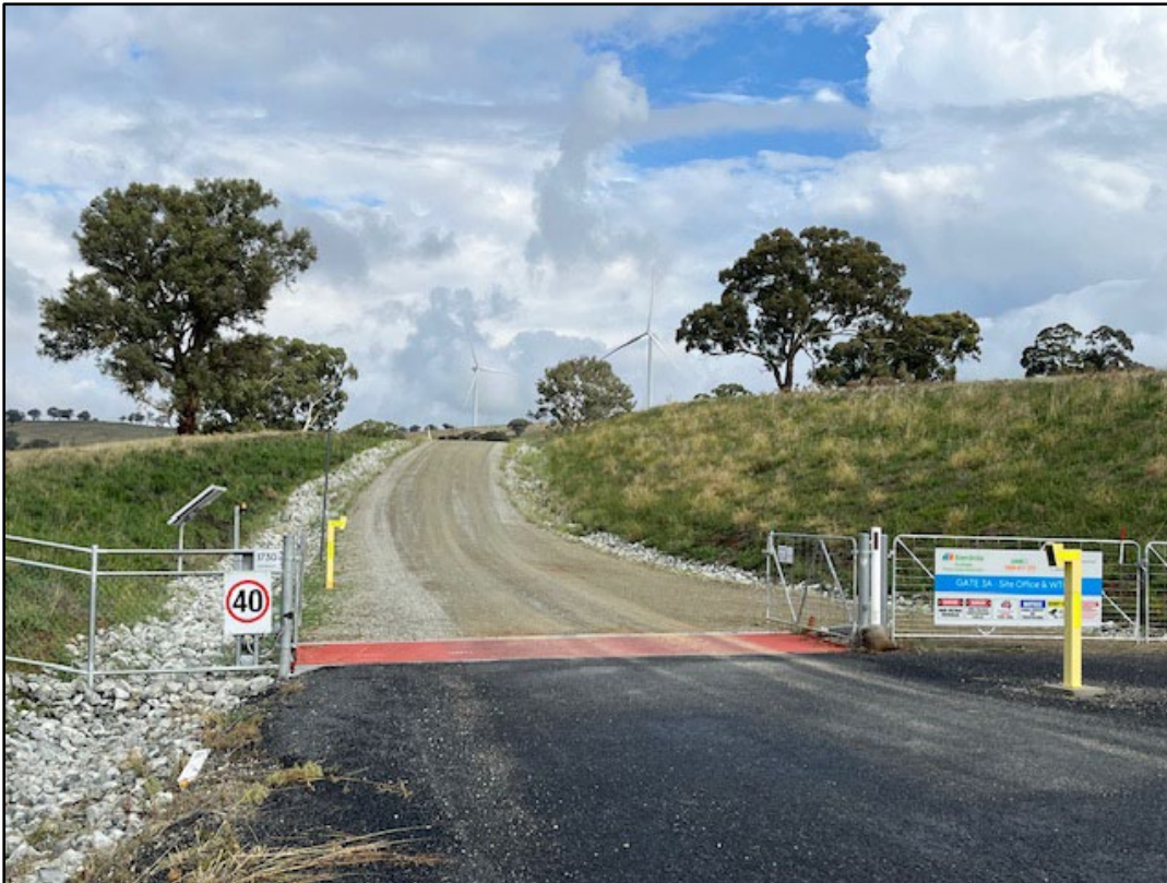
Plate 1: View of signage at the front gate of the Flyers Creek Wind Farm Operations and Maintenance (O&M) Facility showing key project information including contact details. A high standard of landscaping, drainage and road finishing work were noted at the time of the audit site visit.
