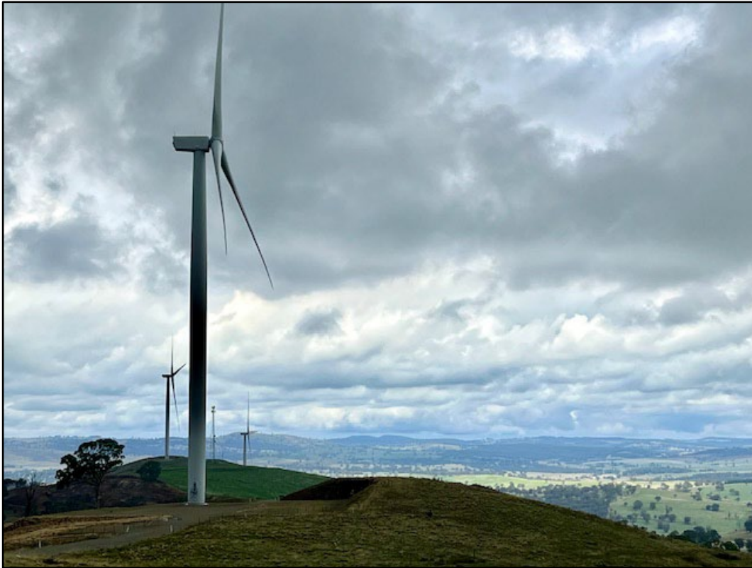
Plate 7: View of turbines 33-35 located to the east of Errowanbang Road. Turbine construction materials were noted to be of low-reflectivity and off-white / pale-grey in colour. Construction areas were very well rehabilitated with good vegetation cover and extensive re-profiling to blend with surrounding
