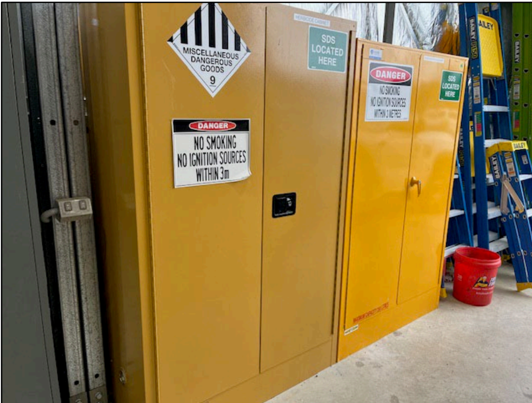
Plate 4: View of a banded Dangerous Good storage cabinets within the O&M Facility. All materials were very well organised and catalogued with SDS's present. Overall house-keeping, procedures and record keeping were of an excellent standard across the site.
