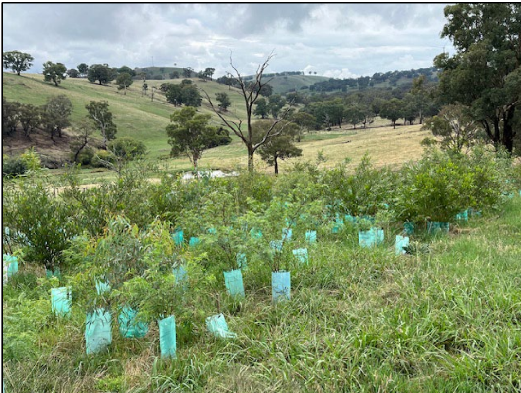
Plate 2: View of site rehabilitation and landscaping works at the site of the O&M Facility at turbines 1-8. Plantings were noted to be healthy and showing vigorous growth. Significant re-profiling, top-soiling and mulching were also evident with resultant excellent rehabilitation outcomes.
