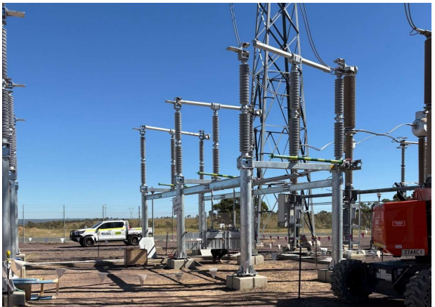
Installation of equipment at Powerlink’s Broadsound Substation
