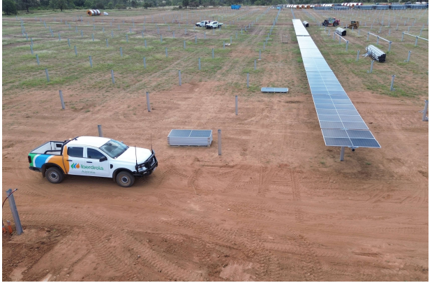
Installation of first solar panels – “Golden Rows”
