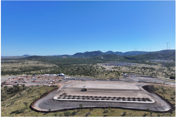
Broadsound Solar Farm Substation and BESS progress
