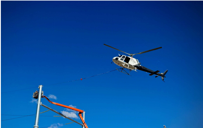
Installation of transmission line conductors
