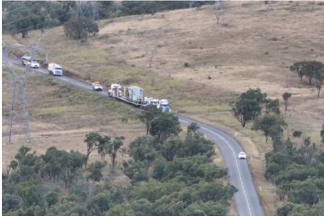
Delivery of Transformer 1
