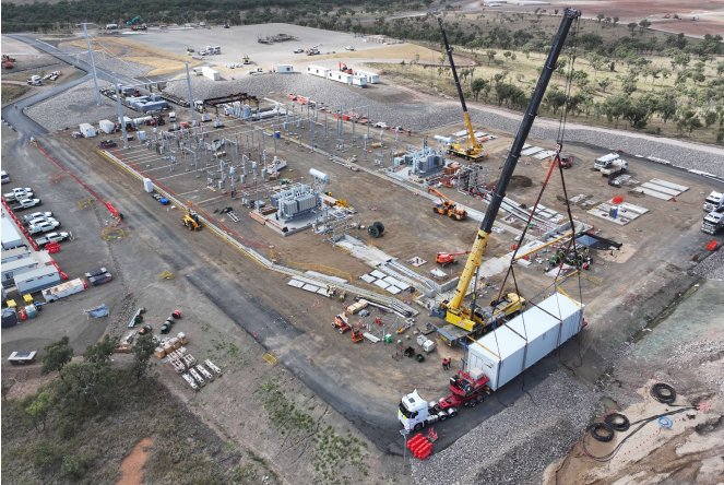
Delivery of Control Building 1
