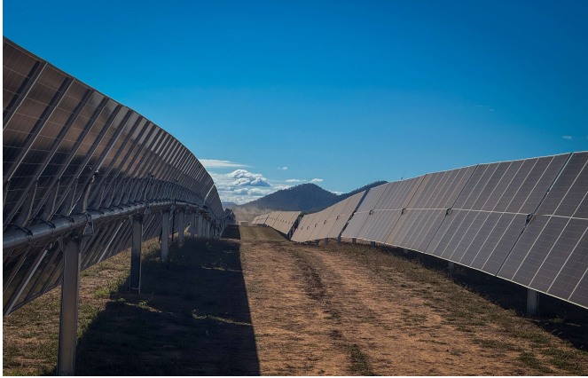
Installation of solar panels
