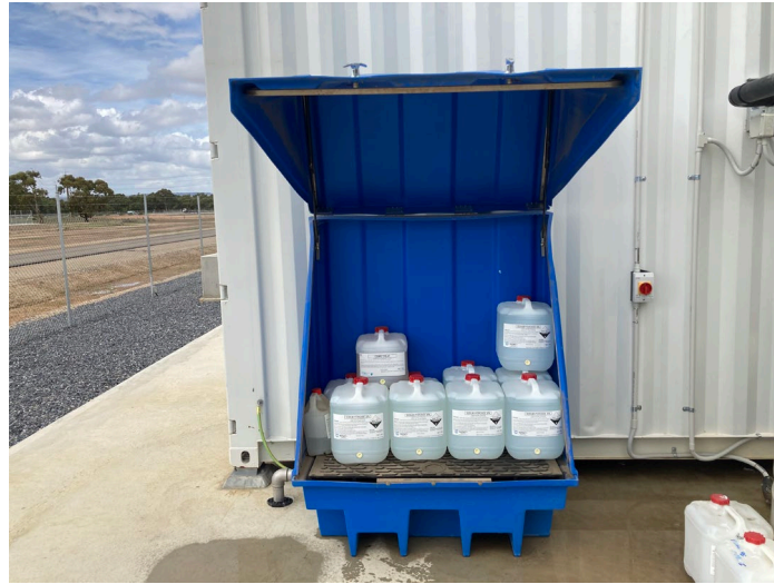
Figure 16: Chemical Storage in Mobile Bunds
