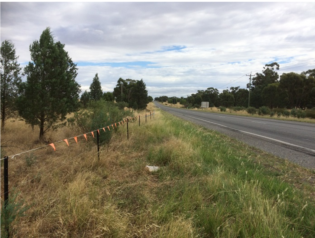
Figure 10-3 Example of exclusion zone fencing.
