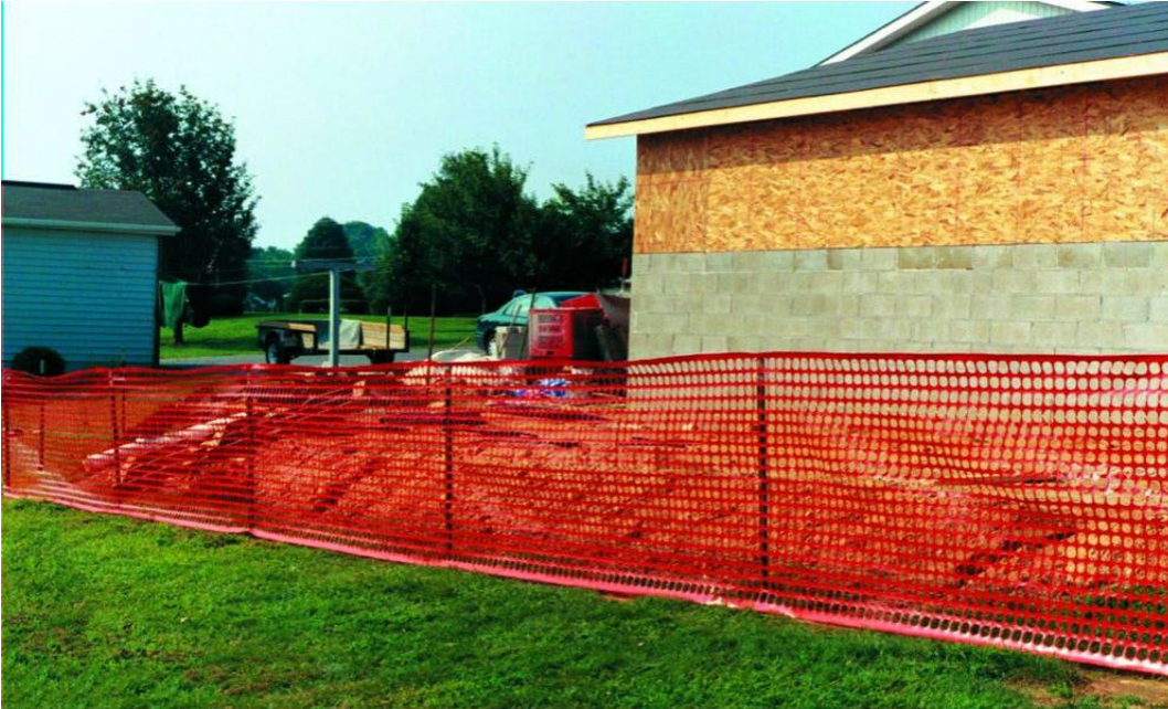
Figure 10-2 Example of para-webbing fencing.
